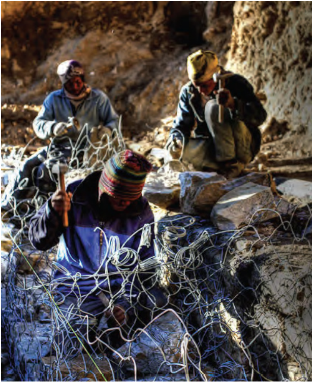
Figure 13. Sherpa villagers weaving seismic cable/wire system into stone wall construction
