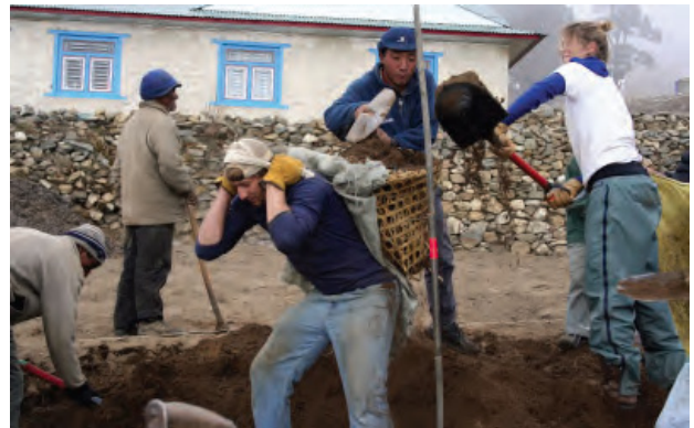
Figure 11. Students and Sherpa working together to excavate for building.
