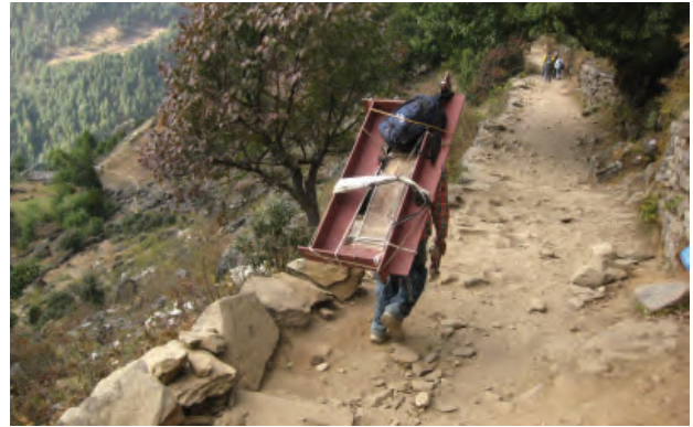
Figure 10. 200 lb seismic brace frame being portered from Lukla to Phortse, Nepal, 2 days per brace frame.
